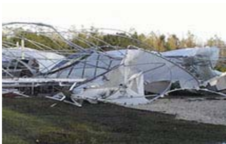
Hydroponics Unit (closeup)
