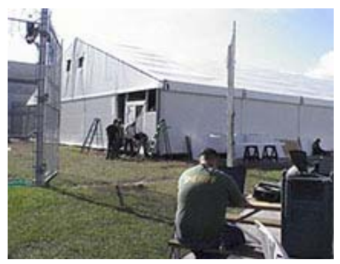
January 31: Building passes final inspection
