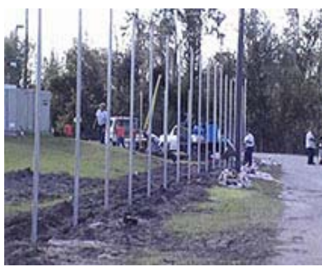
Fence poles being replaced
