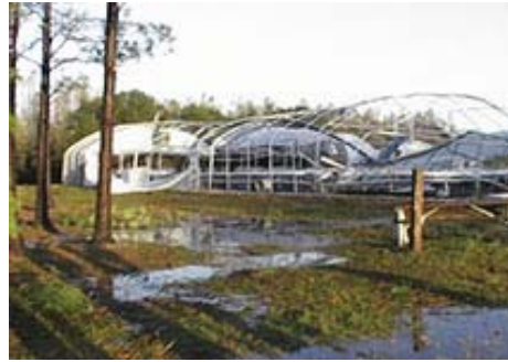
Hydroponics unit destroyed by tornado
